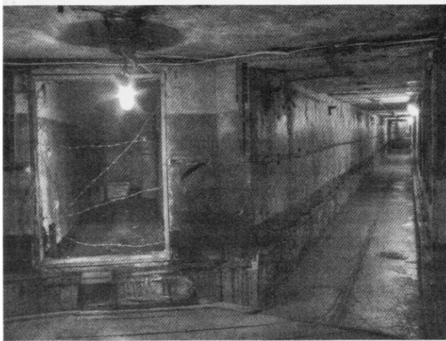
Plokstine R-12U/SS-4 base, corridor to silo. Photo by Tim Robinson
